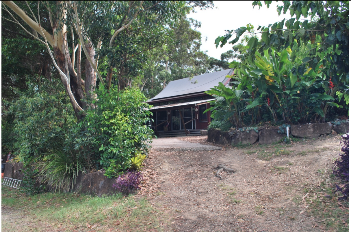
Main group workshop building
